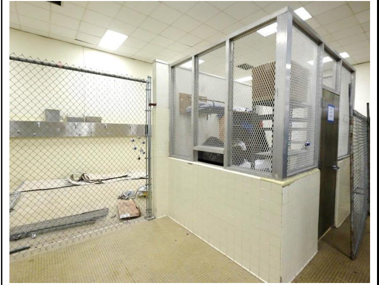
Photo 20 Building Name: Shower/Locker Building Number: 3 Towel room.
