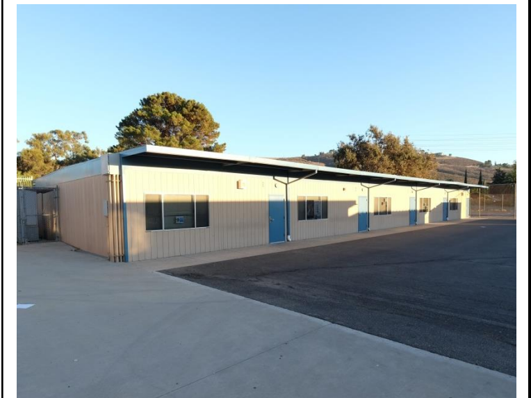
Photo 24 Building Name: Classroom (Modular) Building Number: 9 Basic classrooms .
