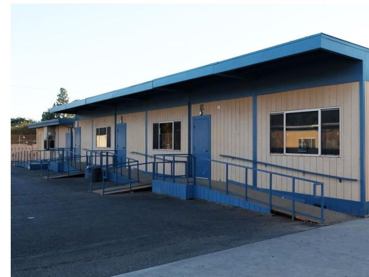
Photo -4 Typical access to portable classrooms.
