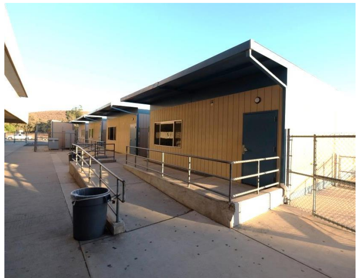
Photo 22 Building Name: Classroom (Modular) Building Number: 5-8 Basic classrooms .
