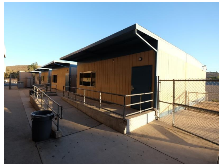
Photo -3 Buildings 5-8 share one ramp to access rooms.
