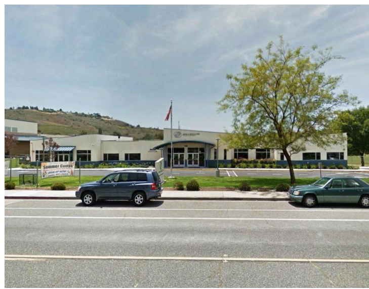
Photo 30 Building Name: Boys & Girls Club Building Number: 11 View from Avenida De Las Flores
