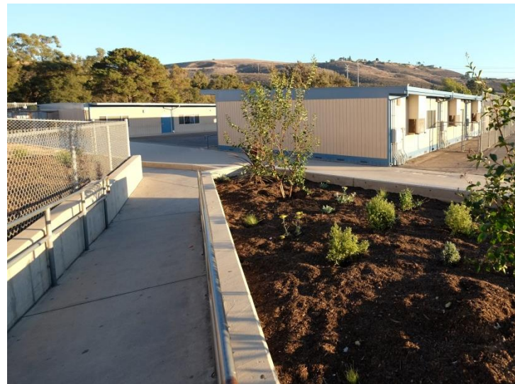
Photo -2 Ramp to lower athletic courts and fields, and Buildings 9 and 10.
